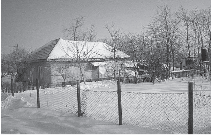
The house built by Andrei and Elena when I conducted my fieldwork. The initial chirpici walls are entirely covered by concrete
